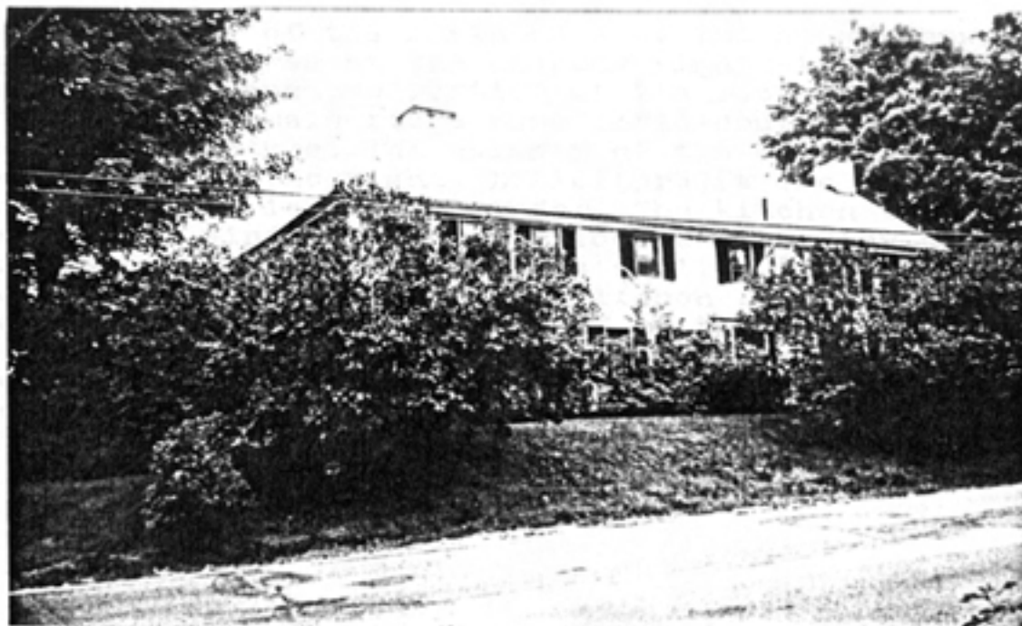
Front View - West Side
